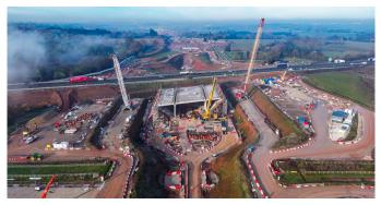
Temporary works specialist, Altrad RMD Kwikform (Altrad RMDK), in partnership with Balfour Beatty VINCI, played a key role in the construction and repositioning of the A46 Kenilworth Bypass Box Structure, a critical element of the HS2 high-speed rail project.
