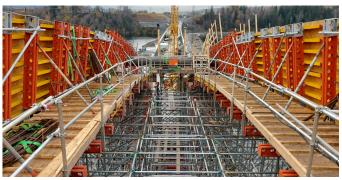
Altrad RMD Kwikform (Altrad RMDK) has supplied a temporary works solution to partner Teknikk AS to aid construction of Minnevika Bridge, the longest railway bridge in Norway, including the creation two vast concrete arches to support the structure.
