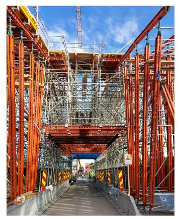
Superslim raking props were used at the ends to accommodate this horizontal load. Ensuring the works could bear the horizontal stresses was crucial to maintain the stability and safety of the construction process.
