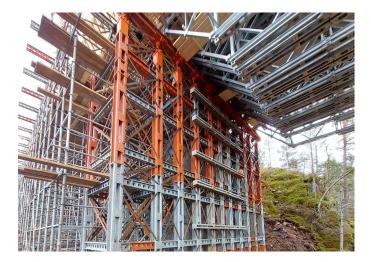
These girders were prefabricated on-site and lifted into position with a large mobile crane.
